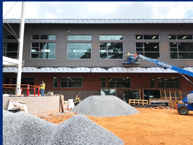
East Wing Metal Paneling Install
