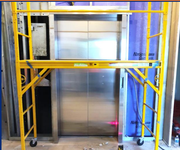
Elevator Door Installation 2 nd Level
