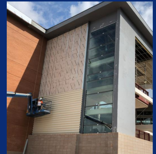
Curtain Wall and Metal Panel Installation South Stair Tower
